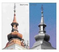
VpCI<sup>TM</sup>-386 Aluminum is non-flammable, UV, and thermal stable; it provides extended corrosion protection in harsh environments. This heavily corroded and weathered church roof was restored with VpCI<sup>TM</sup>-386 Aluminum.
